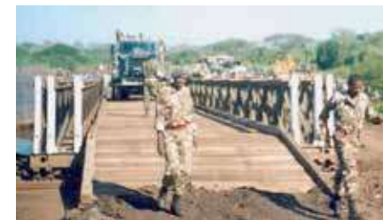
Fig 1 – Thange Bridge jacked down across the gap
